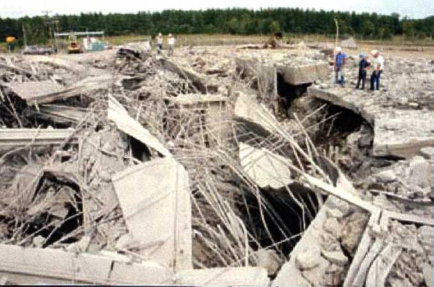
Workers examine shattered concrete and twisted wire at a destroyed Titan II missile silo in Arkansas, 1987.
